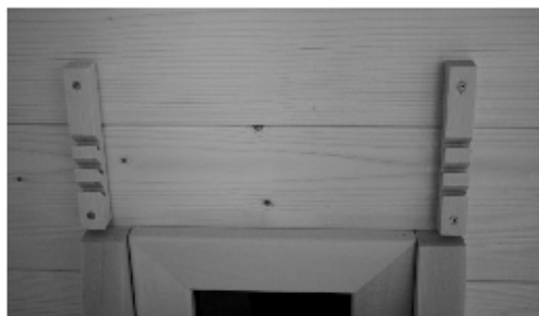
Fig. 47: Installation of the headrests
