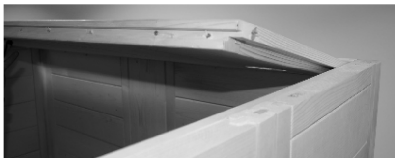
Fig. 17: Installing the roof element in the front
