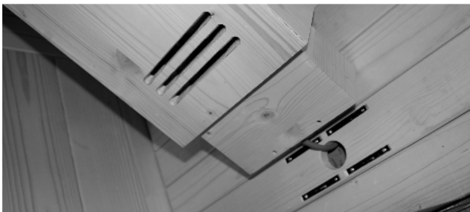
Fig. 27: Attach the front radiator in place
