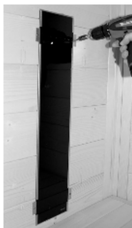
Fig. 36: Install the rear radiator (infrared radiator ECO 350)
