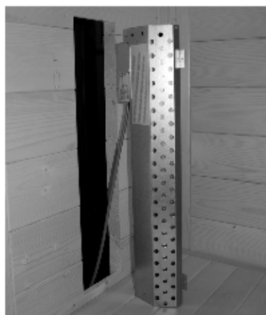
Fig. 36: Install the rear radiator (infrared radiator ECO 350)
