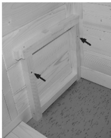
Fig. 30: Installation of the bench cushion
