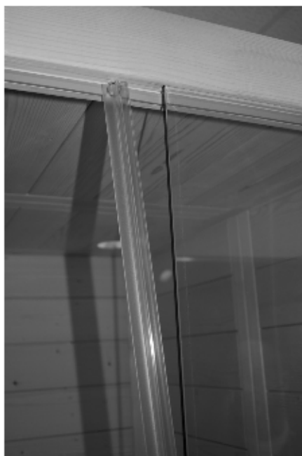
Fig. 19: Installing the door insulation strips
