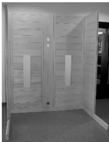
Fig. 7: Pre-assembled rear wall
