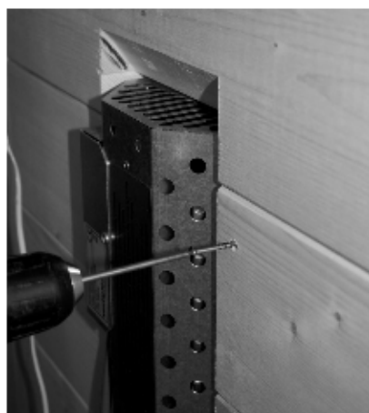
Fig. 37: Installing the rear radiator blind
