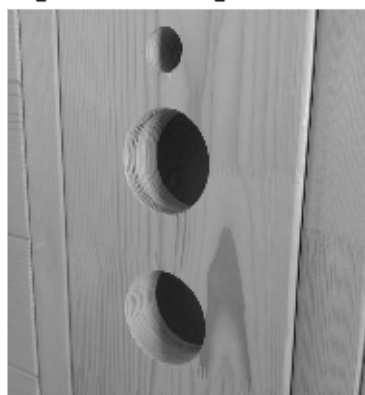
Fig. 43: Installing the control panel
