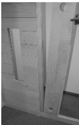
Fig. 6: Install the electrical element in place
