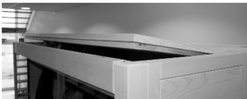
Fig. 17: Installing the roof element in the front
