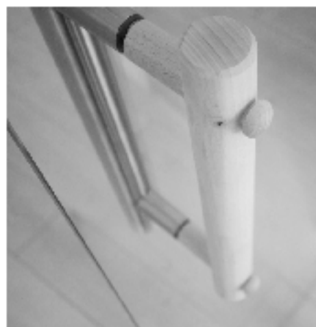
Insert silicone ring in the drill holes
